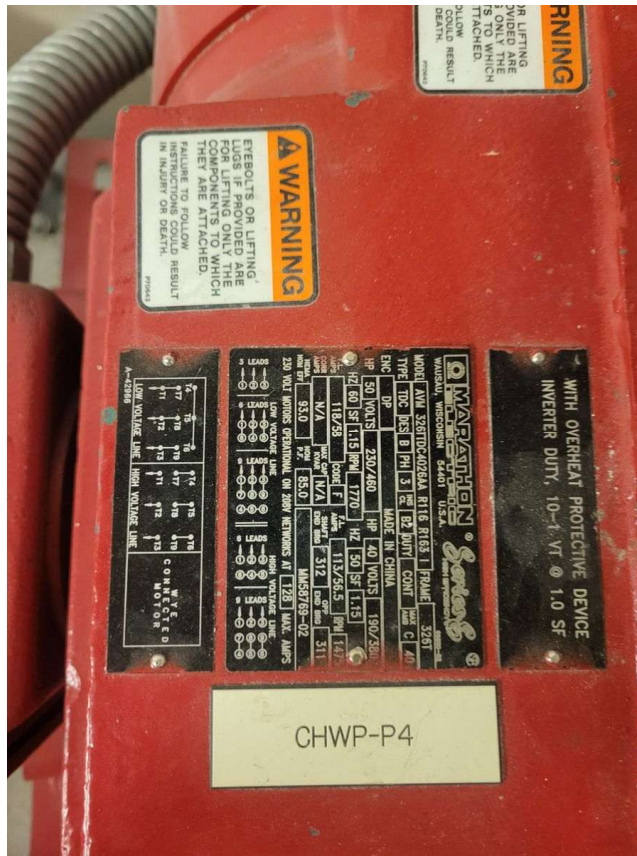
Photo A.3b — CHWP-P4 drive motor (Marathon/Emerson, 50 HP, 460V, 3-phase). Inverter duty rated. Chilled water pump P4 identification tag visible.
