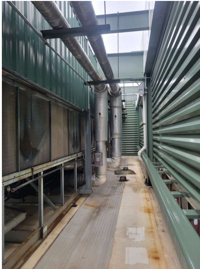
Photo A.1b — Pit corridor looking north. Large insulated chilled water supply and return headers run overhead within the pit. The pit enclosure walls are visible above, limiting condenser discharge height.
