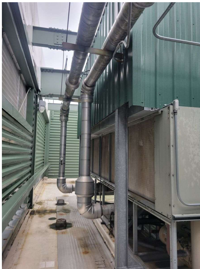
Photo A.1b — Pit corridor looking north. Large insulated chilled water supply and return headers run overhead within the pit. The pit enclosure walls are visible above, limiting condenser discharge height.
