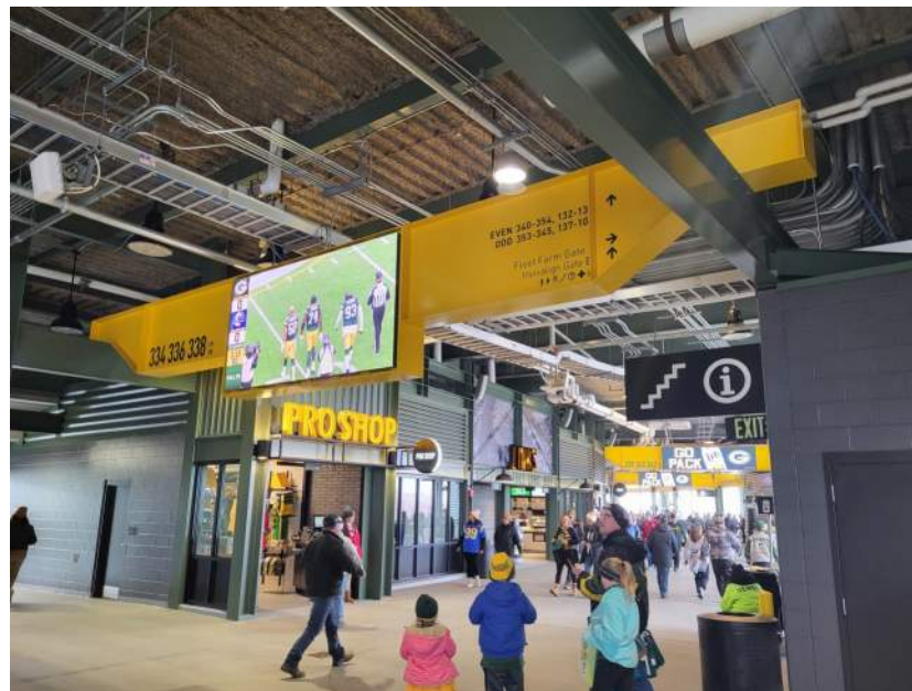
Photo 14: 300 concourse signs and screens
