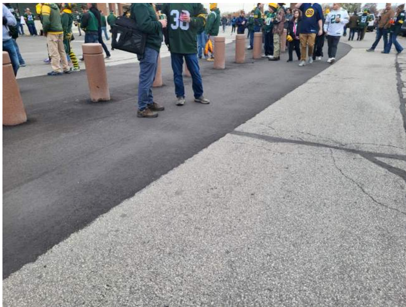
Photo 6: Replaced asphalt along barricade perimeter
