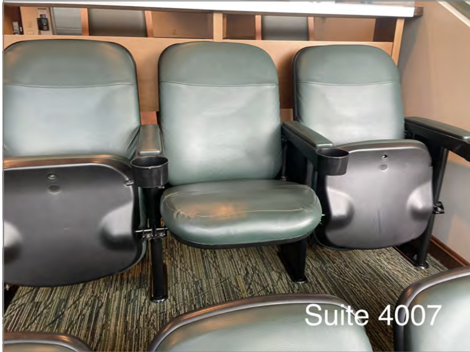
Interior and Finishes: Photo 4-4-25 Chair seat does not automatically close
