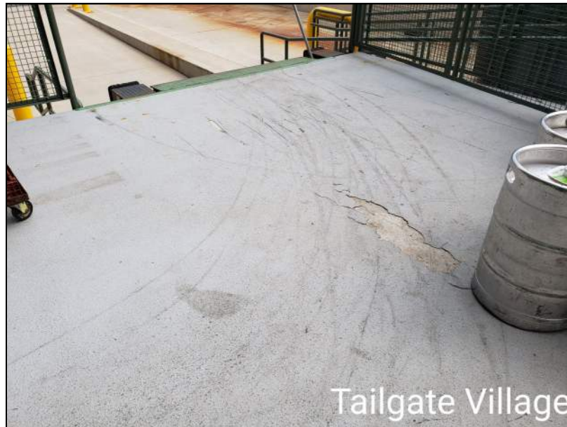
Site: Photo 10-1-3 Traction Coating Damage
