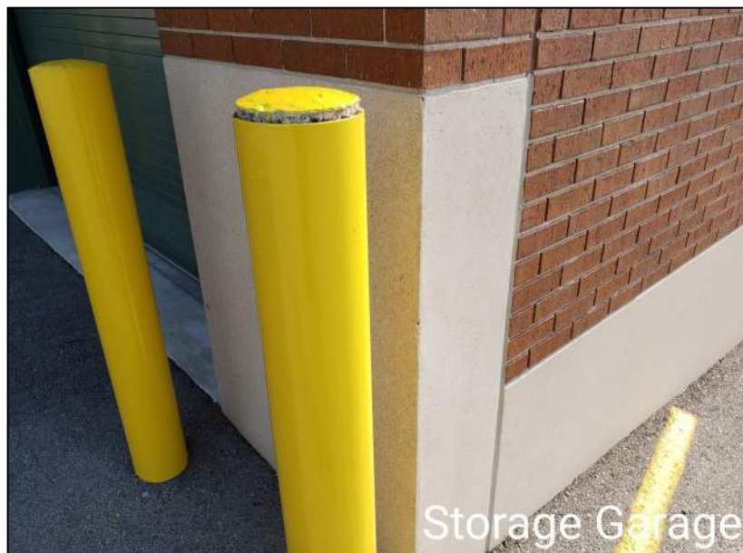
Site: Photo 10--7 Bollard Settling
